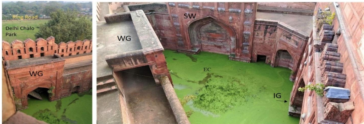
Figure 7: Two stitched photos showing Inside view from terrace of Asad Burj: Barbican enclosing external courtyard (EC) having two outer and one inner gate. Water Gate (WG) facing Delhi Chalo Park and Ring Road; Inner Gate (IG) towards inner Water tank; South West (SW) facing outer gate with no name
