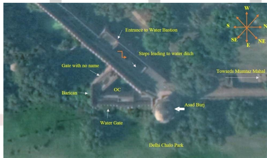
Figure 2: Google earth 3D view of south east corner of Red fort. Barican enclosing triangular outer courtyard (OC).
