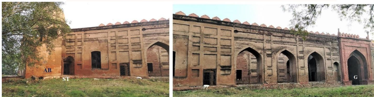
Figure 6. Terrace view of Asad Burj
