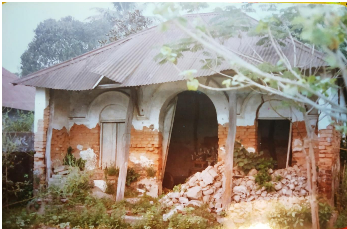
Fig.-10: Durga Mandap at the house of Govinda Prasad Roy, 1992 C.E.; this tin-roofed pucca building represents the typical rain-frequented, earthquake-prone ‘Cooch Behar typology’ (courtesy: Shree Ramashish Roy, Delhi).
