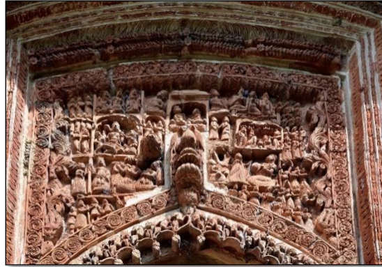
Fig.1: Construction between 1 st and 2 nd arches
