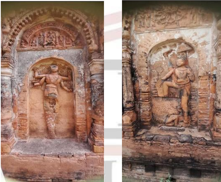
Fig. 3: Damaged Matsyavatara(left) and Vamanaatara(right) at Ratneswar temple: Bhattabati
